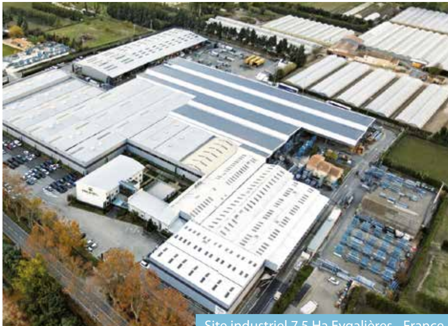
Site industriel 7.5 Ha Eygalières - France
